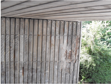
Corrosion of reinforcement due to leaking joints and spray from passing traffic, chloride contamination a major issue
