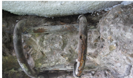
Corrosion of reinforcement due to leaking joints and chloride contamination are a major issue
