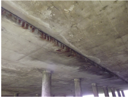
Corrosion of reinforcement due to leaking joints and chloride contamination are a major issue
